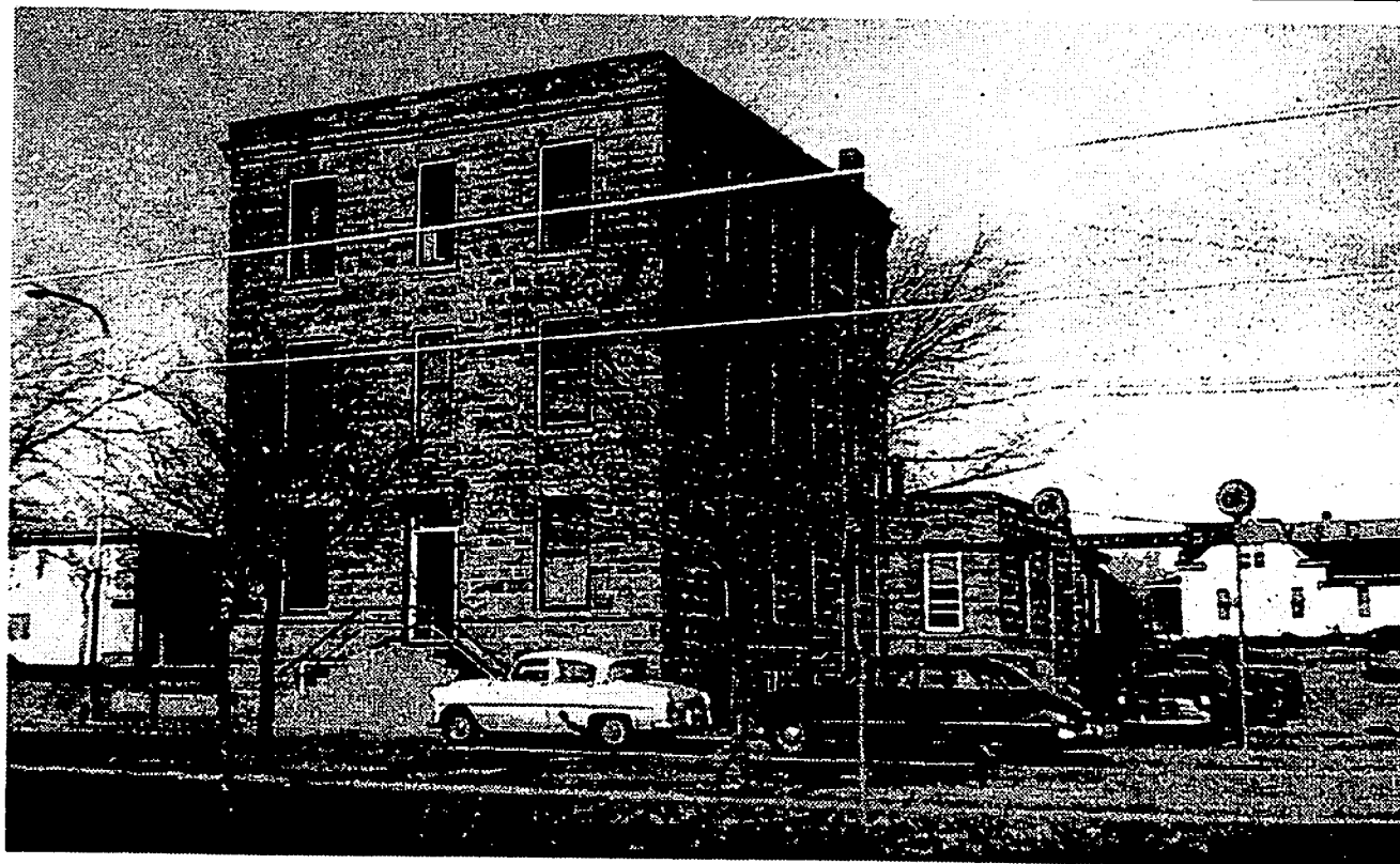
This photo was provided by Bob and Rose Fettig, and it shows south side of the Stone Apartments from the east side of Fettig's yard. The photo was taken in the late 1950's. Notice the one-level addition, and the V & C Motors car lot to the right. Plus Volk, who co-owned the car dealership and the apartment complex, lived in one of the two apartments in the addition, while the other was used as an office for the business. Also notice the two-story home in the background. It is located where the Linton Post Office now stands.
